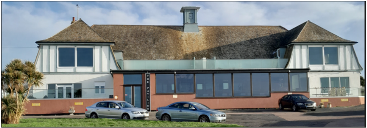
Image 9: south western elevation with first floor balustrade
